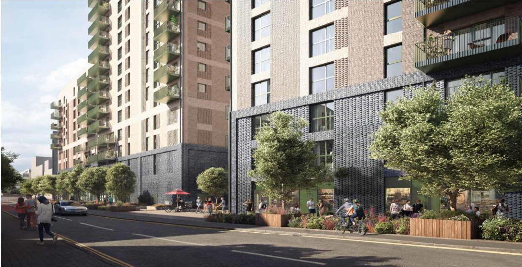
View Along Market St.
